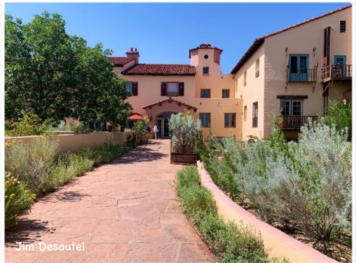
Walkway into the Hotel & Restaurant
