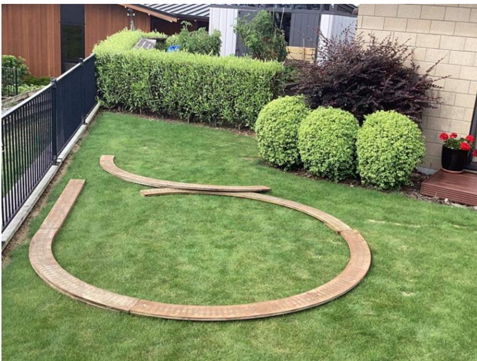
From here the tracks separated on to 18mm plywood road beds to the reverse curve.
