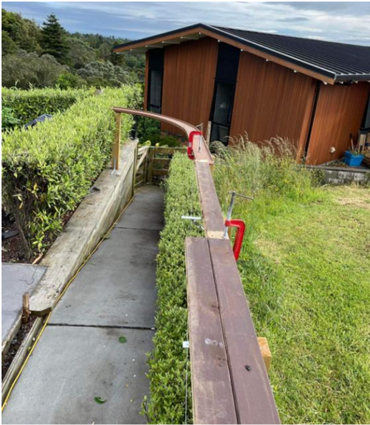
The LH curve was recycled from Auckland. The two mains will be reduced to a single line for the curve with a RH set of points.
