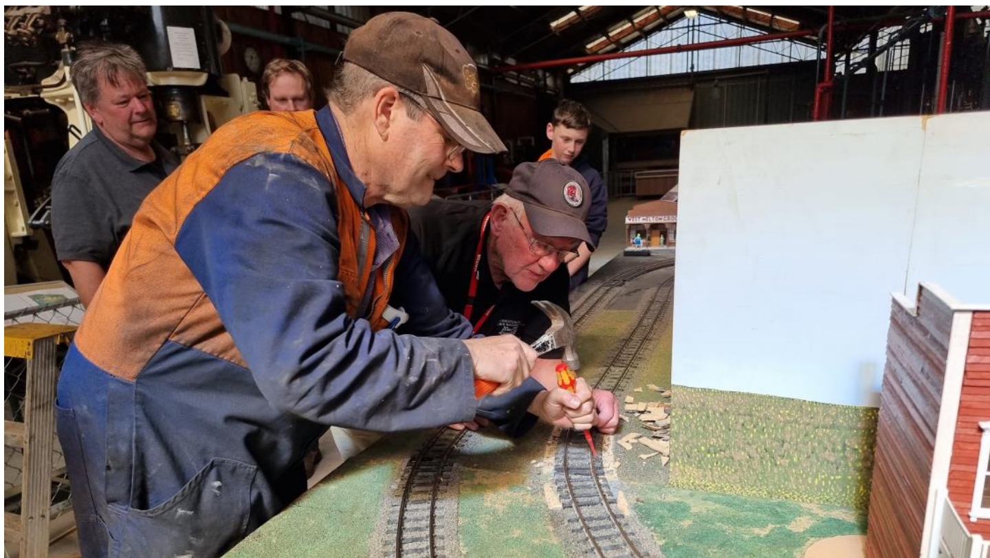
Repairs to the club layout track - Photo Bill Stanley.
