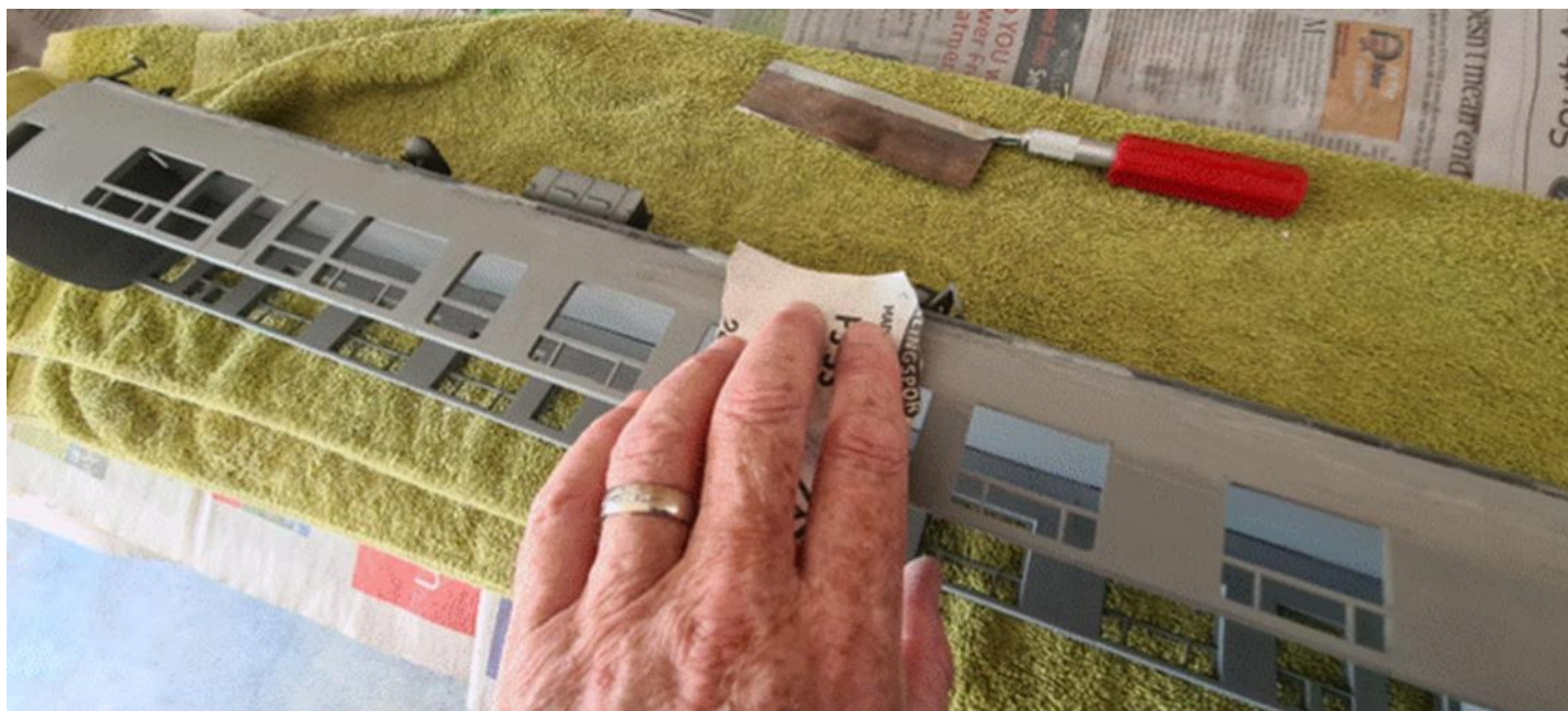
Rubbing down the first primer coat.
