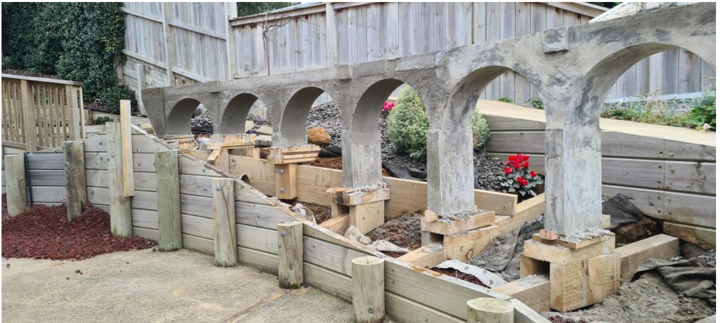
These were the last of the refuges and therefore the last part of the viaduct to be cast. Formwork has been removed.
