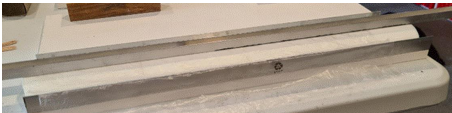
Aluminium channel placed on the crown of the roof
