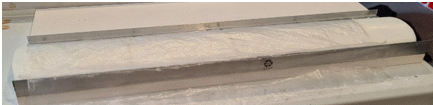
Roof assembly jig with polythene film placed over it.
